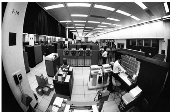
now comprised five linked **IBM 7094s**, five **IBM 2361 Core Storage Units**, and two **IBM 1460s**. The **IBM 2361** was the largest computer memory ever built by the company and consisted of nearly **20 million doughnut-shaped ferrite cores**, capable of storing 2.6 megabytes of data.
